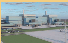
Bison Gen. Station Epping, N.D. • 2030 1,490 MW • Nat. Gas
