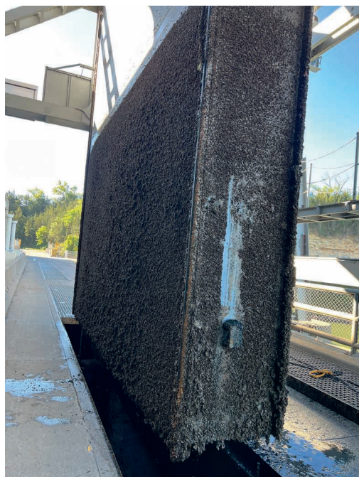
Zebra Mussels completely envelop Gavins Point Dam's water gates, adding up to an additional 30 tons of weight.
